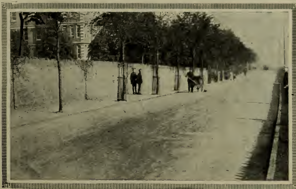
MAIN ROAD FROM NEWPORT AND CARDIFF: CONSTRUCTED OF CONCRETE WITH "B.R.C." FABRIC REINFORCEMENT.
